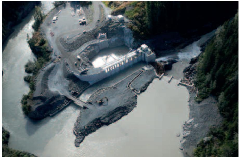
Figure 6 - Intake facility that includes field monitoring sensors, sediment sluicing facilities and a desander
