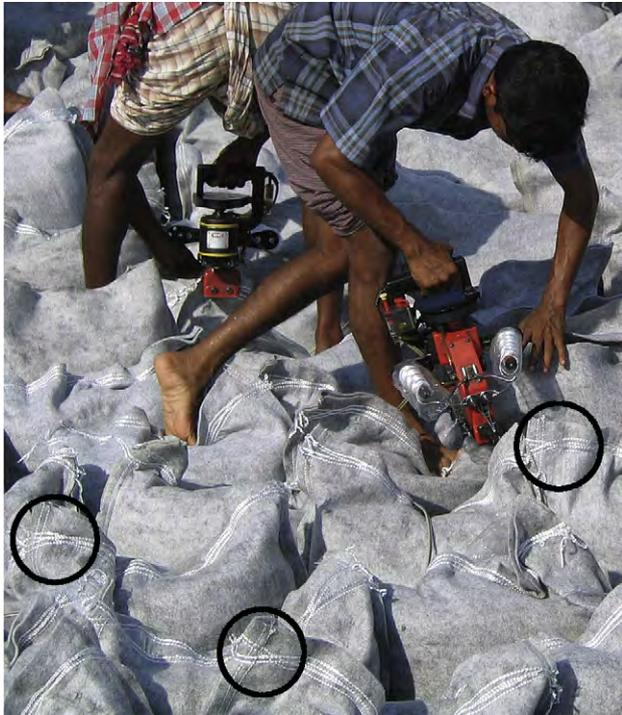
Fig. 3. Closing bags at the site with two lines of type 201 seam.
