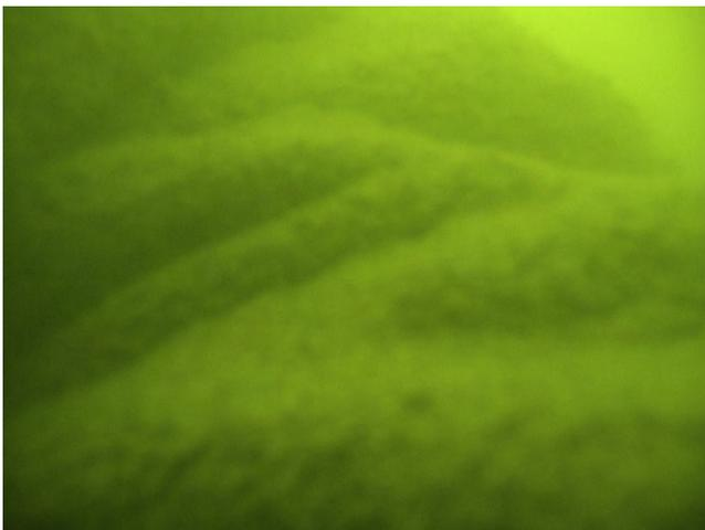
Fig. 17. Observed undulations of geotextile bag surface under water.
