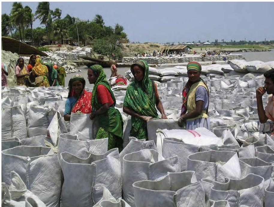
**Fig. 2.** Filling of geotextile bags.
