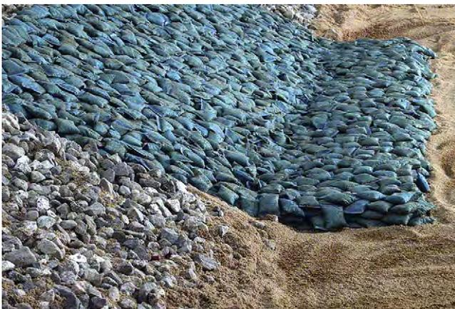
Fig. 8. Model of lower bank slope with initially installed falling apron.
